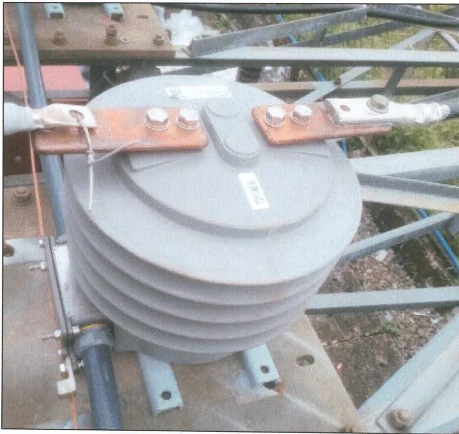
Item no. 12. Transformer, current transformer, outdoor, 600:5
