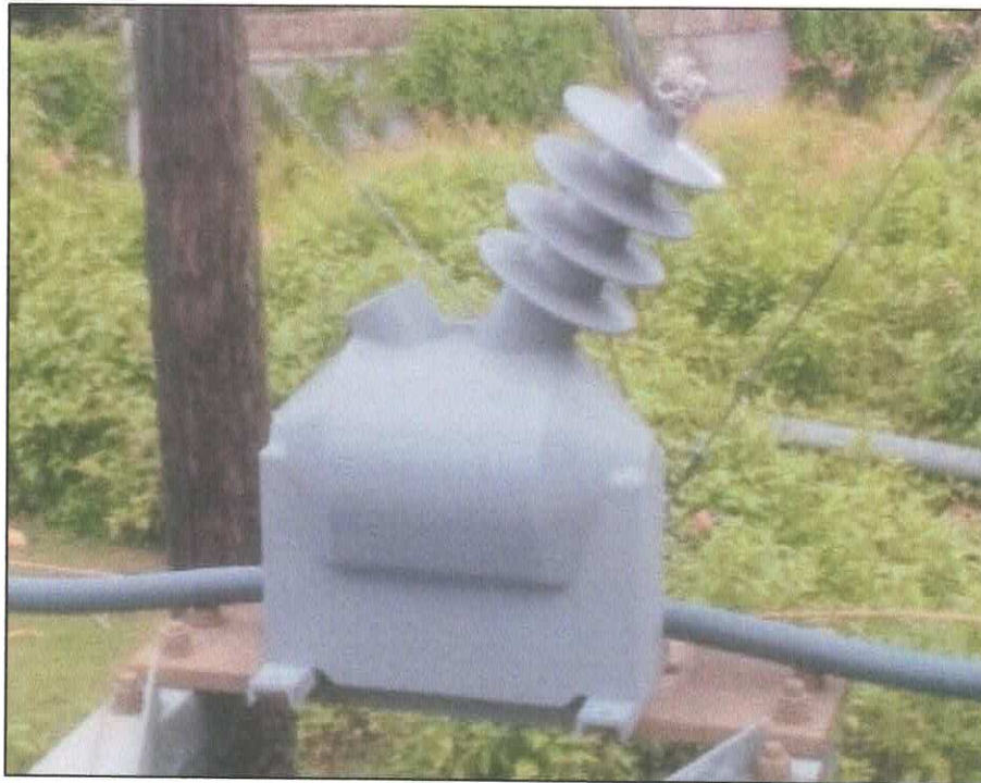
Item no. 13. Transformer, voltage transformer, outdoor
